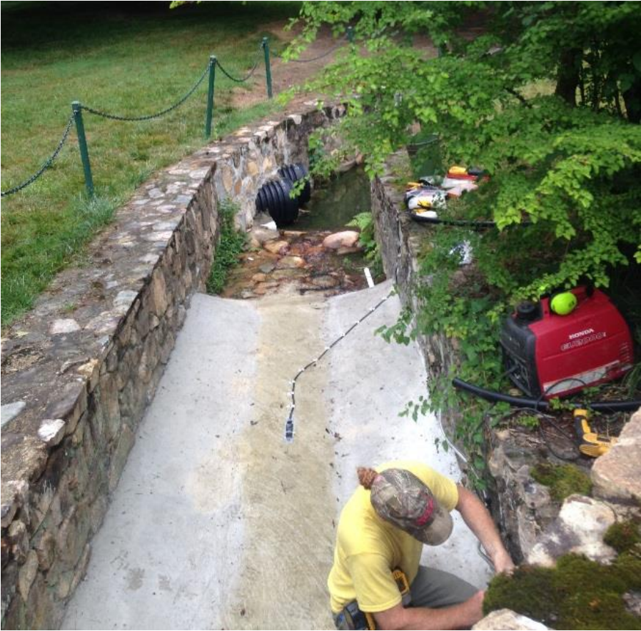
Figure 5. NCSU staff installing monitoring equipment at the site.
