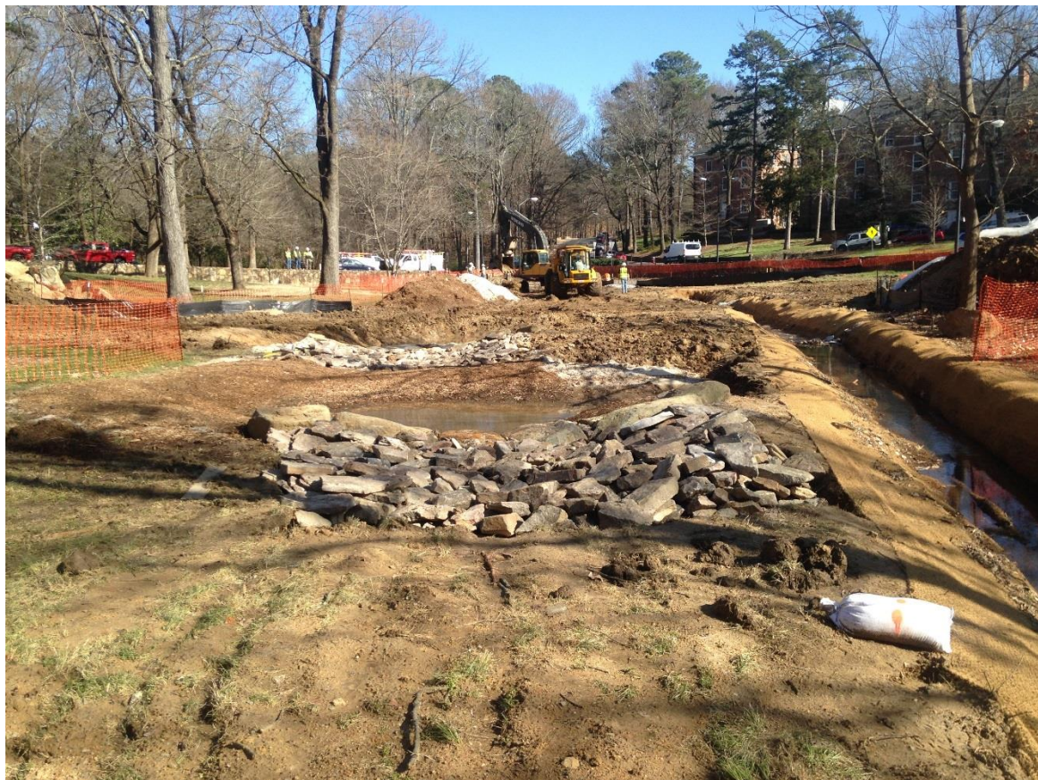
Figure 3. While the pool and riffle complex was constructed, the stream was routed through a side-channel.
